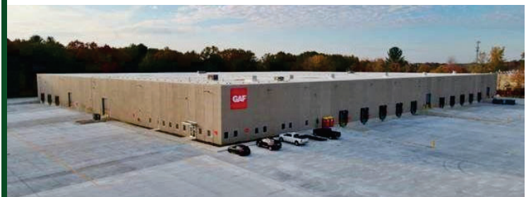
200,000 SF GAF Materials building in Michigan City
